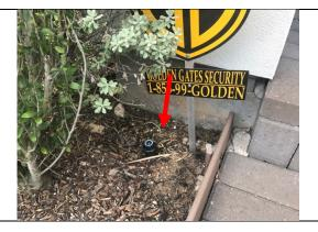
Sprinkler heads are in close proximity to the stucco walls. It is recommended to re-direct all sprinkler heads away from stucco walls
