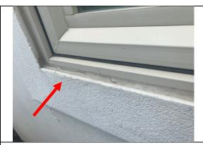
Sealants at all stucco- window junctions have reached their life expectancy. Sealants are starting to fail adhesively and cohesively It is suggested to have all sealants replaced every 2-3 years
