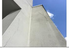
Hairline cracking noted in several locations. Suggested to seal/paint cracks throughout. Any thicker cracks should be grinded out and retextured.
