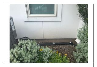
Light mildew/run-off staining noted along base of stucco wall.
