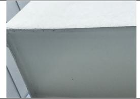
Stucco overhangs noted to terminate with a perforated casing. Many holes along the casing, however, have been covered with paint/stucco materials. Suggested to re-open
