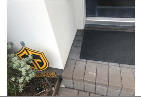
Stucco walls noted to have a proper clearance from the floor. The stucco terminates with a weep screed. This is favorable. The entry pavers, however, are brought up to the base of the stucco walls.
