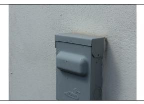
All penetrations through the stucco are lacking a quality, low modulus sealant, needed for **long lasting** protection against moisture intrusion
